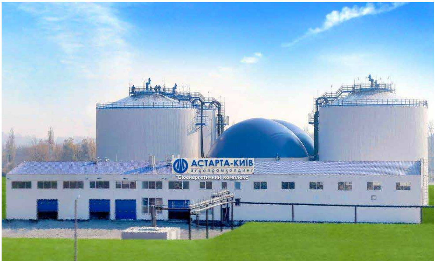
Figure 8 Globyno biogas plant
